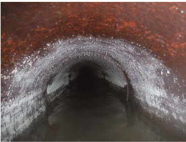
North Influent Pipe
