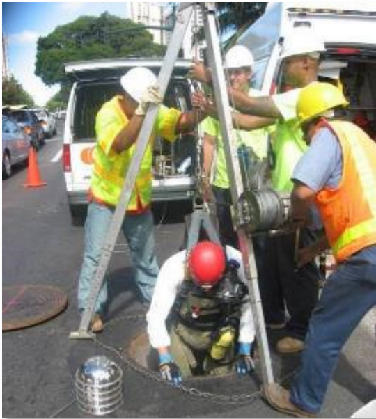
Photo 2-1. Confined Space Entry
