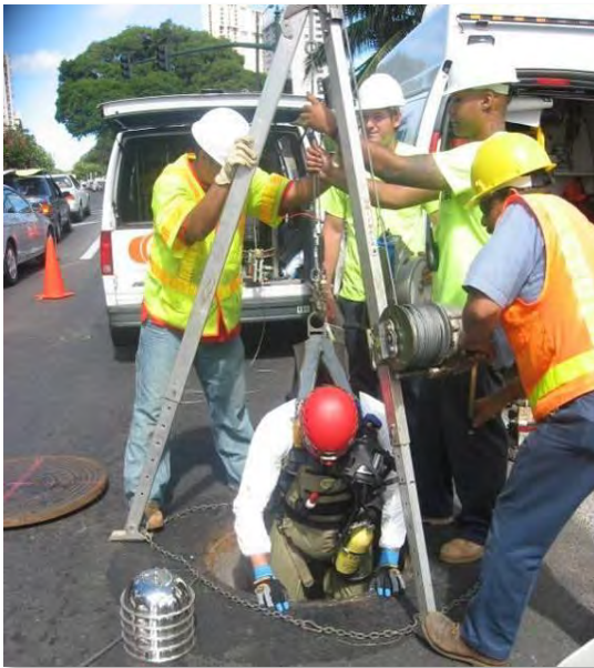
Photo 2-1. Confined Space Entry
